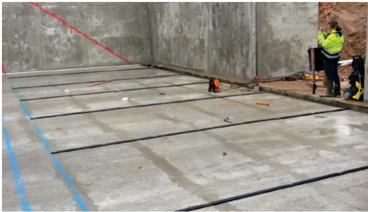
Figure 18. Rubber ribs for sectioning of seepage water during downstream support fill. The flow measured with Thomson weirs (Bernstone et al., 2021).
