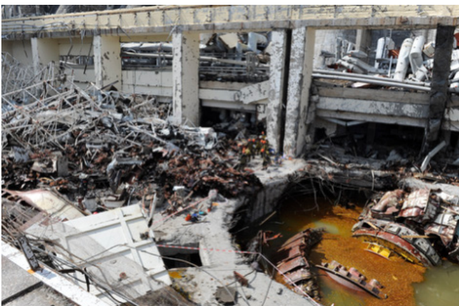
Figure 1: Severe failure at Sayano-Shushenskaya power station 2009.
